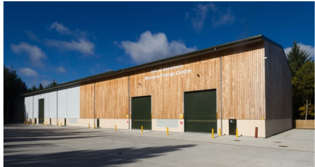
Figure A2.4 Biomass centre with wooden cladding
