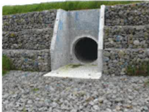
Typical RENO Mattress installation
