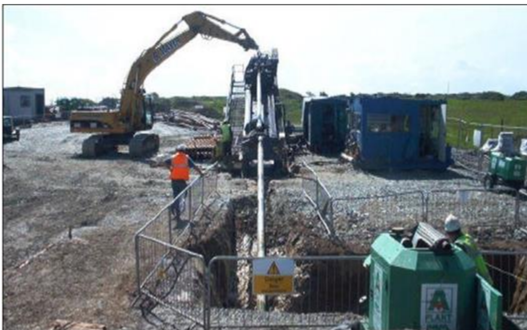
Figure 20: Illustrative visualisation of a landfall HDD Installation.
