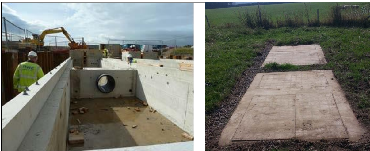
Figure 18: Typical Transition Joint Bay during construction (left) and two link boxes, each with manholes for electrical and optical cable joints, after reinstatement (right) (courtesy of RWE renewables UK Ltd).
