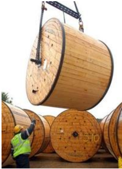
Figure 26: Example of a cable drum delivery to cable storage area (Courtesy of Scira Offshore Energy).
