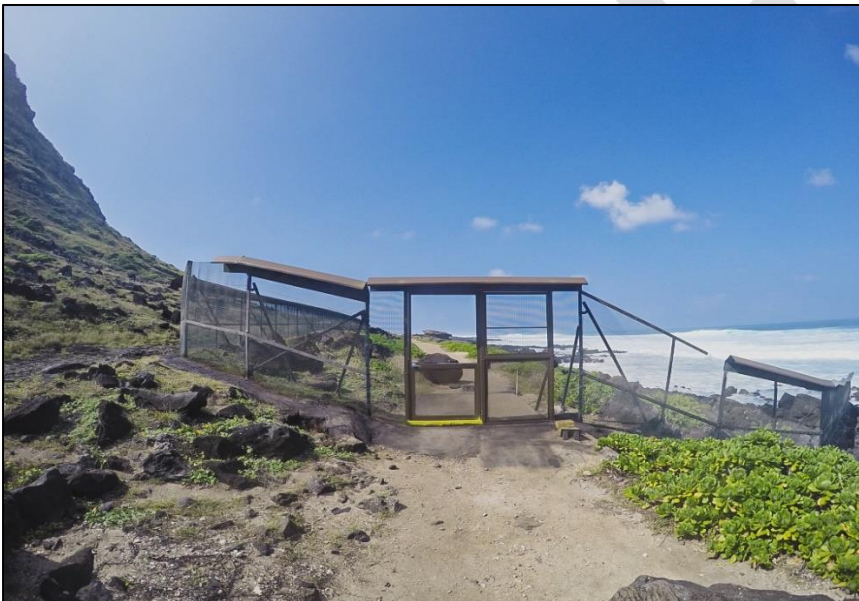
Image 78. Example of an access gate on a predator-proof fence.
