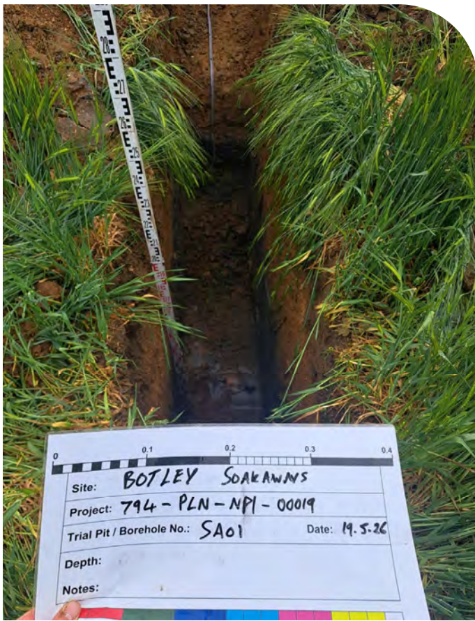
Photo 1: View of SA01 Test Pit.
