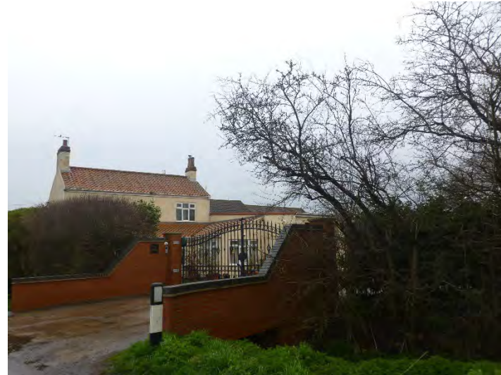
Plate 57: View of The Willows, looking north-east
