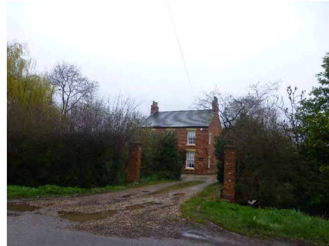
Plate 55: View of Meaburns, looking east
