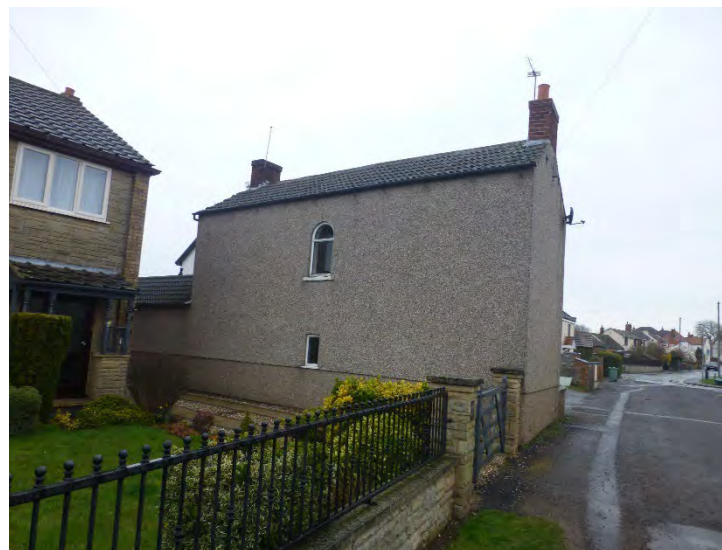
Plate 33: View of 6 Marsh Road looking east
