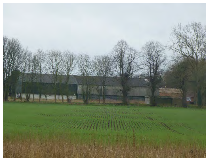
Plate 36: View of Belton Grange looking south
