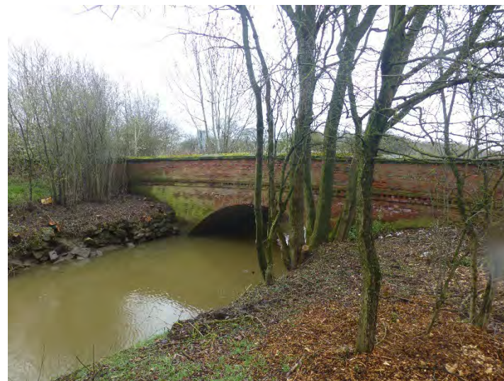
Plate 22: View of bridge adjacent to Dirtness Cottage
