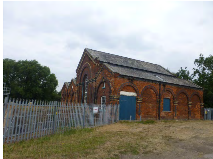
Plate 27: View of Dirtiness Pumping Station looking north-east
