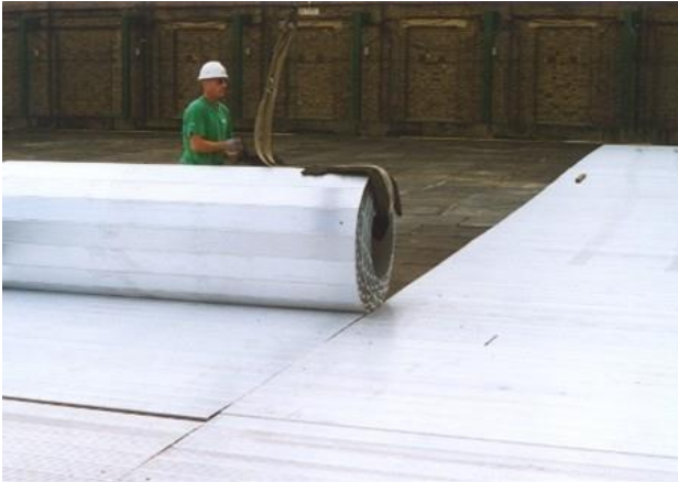
Light Duty Trakway being rolled out.
