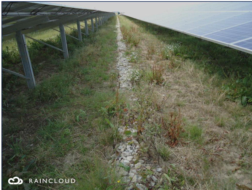
Plate A9.1.43: Example filter drains at solar farms
