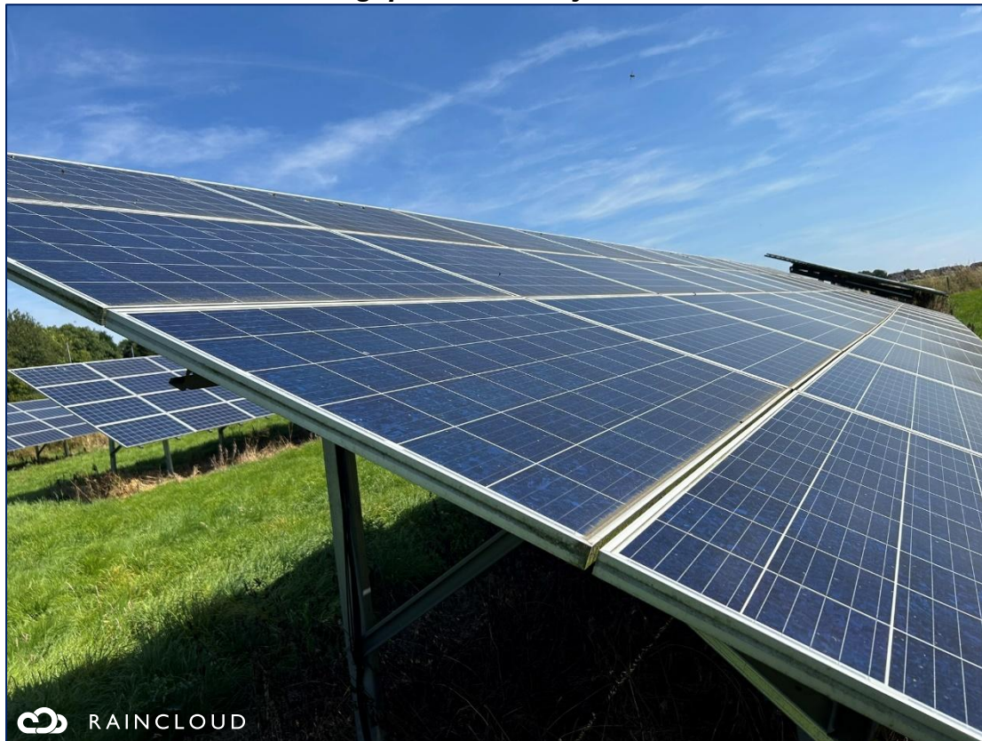
Plate A9.1.37: Rainwater gaps on PV array table
