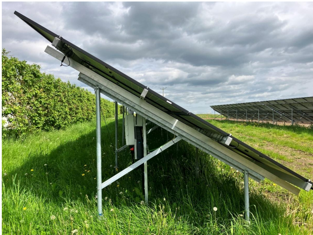
Plate 9.20 Typical thin Mounting System driven into ground
