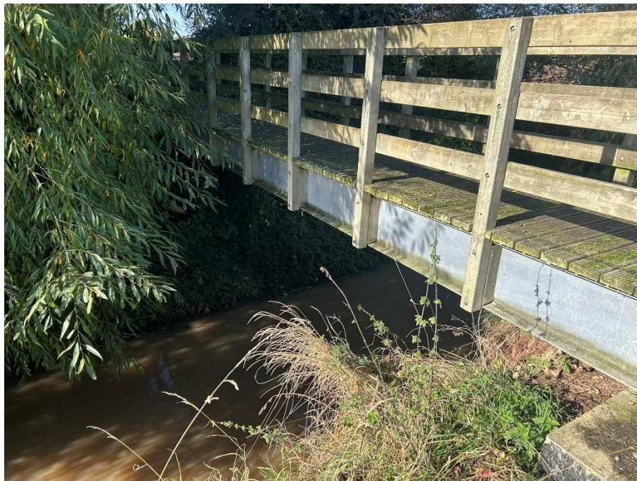
Plate 9.6: Beam deck bridge over Moorhouse Beck
