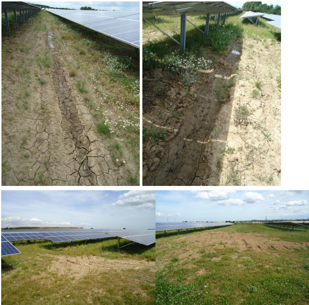
Plate 9.24: Poor practice vegetation establishment examples on solar sites
