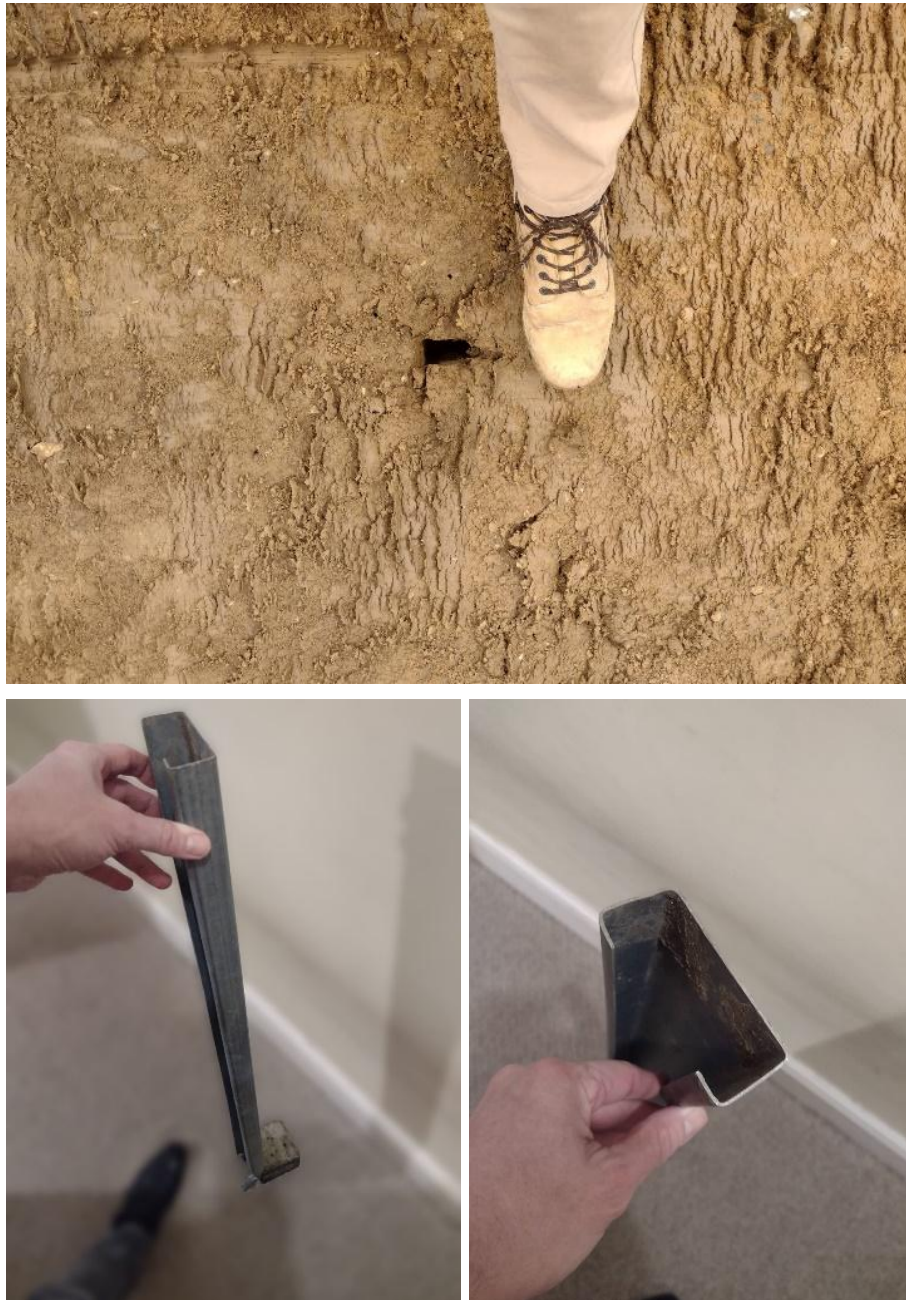
Plate 9.19: PV mounting pile and physical footprint 49
