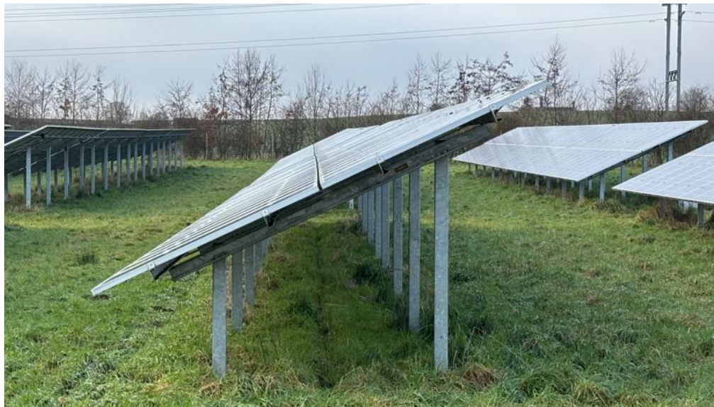
Plate 9.23: Operational solar farm with established vegetation and drip lines
