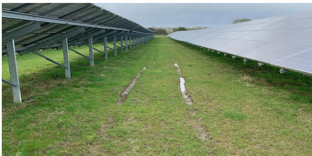
Photo 17.44: Example of Minor Ruts Caused by Vehicles
