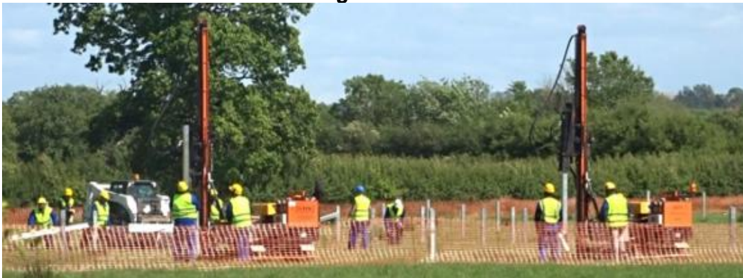
Photo 17.37: Framework Piles being Installed
