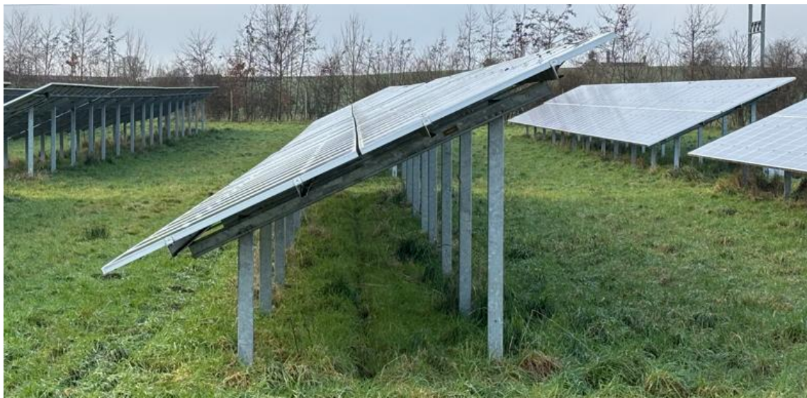
Photo 17.46: Panels Array Showing Gaps Between Panels
