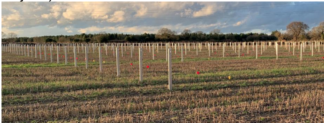
Photo 17.38: Framework Posts being Installed (taken at Tiln Farm, Retford, in January 2023)
