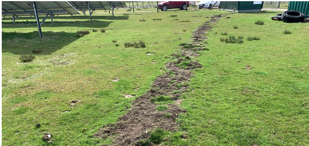
Photo 17.45: Emergency Trench Installed During Wet Period
