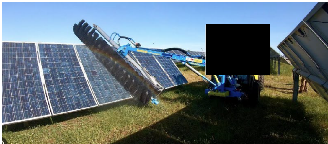
Photo 15.20: Cleaning of Solar Modules
