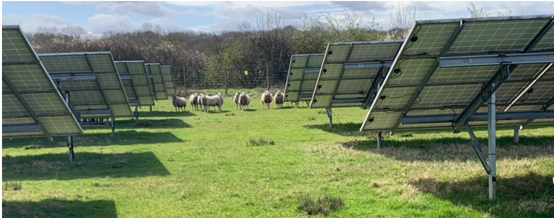
Photo 15.24: Grass Growth Below and Between Arrays
