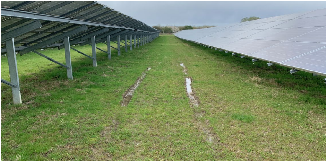
Photo 15.21: Example of Minor Ruts Caused by Vehicles
