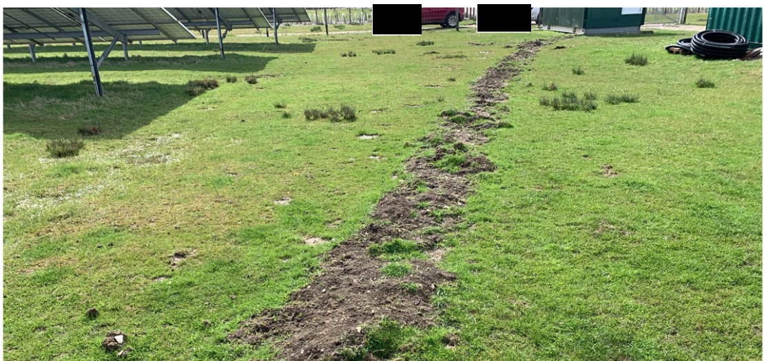
Photo 15.22: Trench During Wet Period
