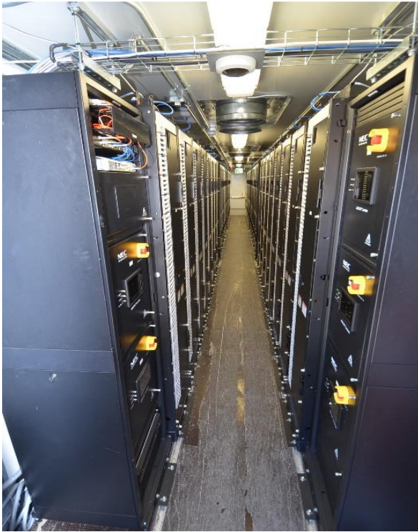
Image left: Central internal view of unaffected unit. Note configuration of lithium ion banks and narrow access corridor.
