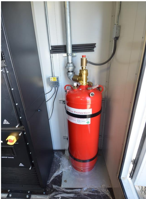
Image left: NOVEC 1230 fixed aerosol system with piping.
