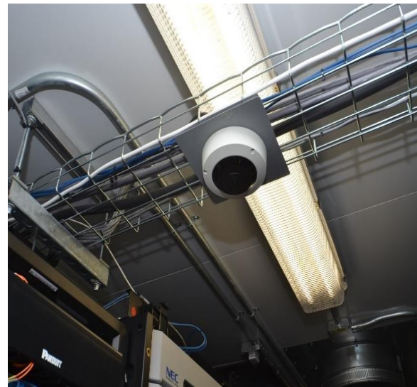
Image left: NOVEC 1230 fixed aerosol system with piping.
