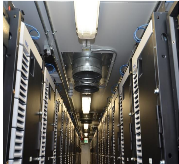
Image left: Central internal view of unaffected unit. Note configuration of lithium ion banks and narrow access corridor.
