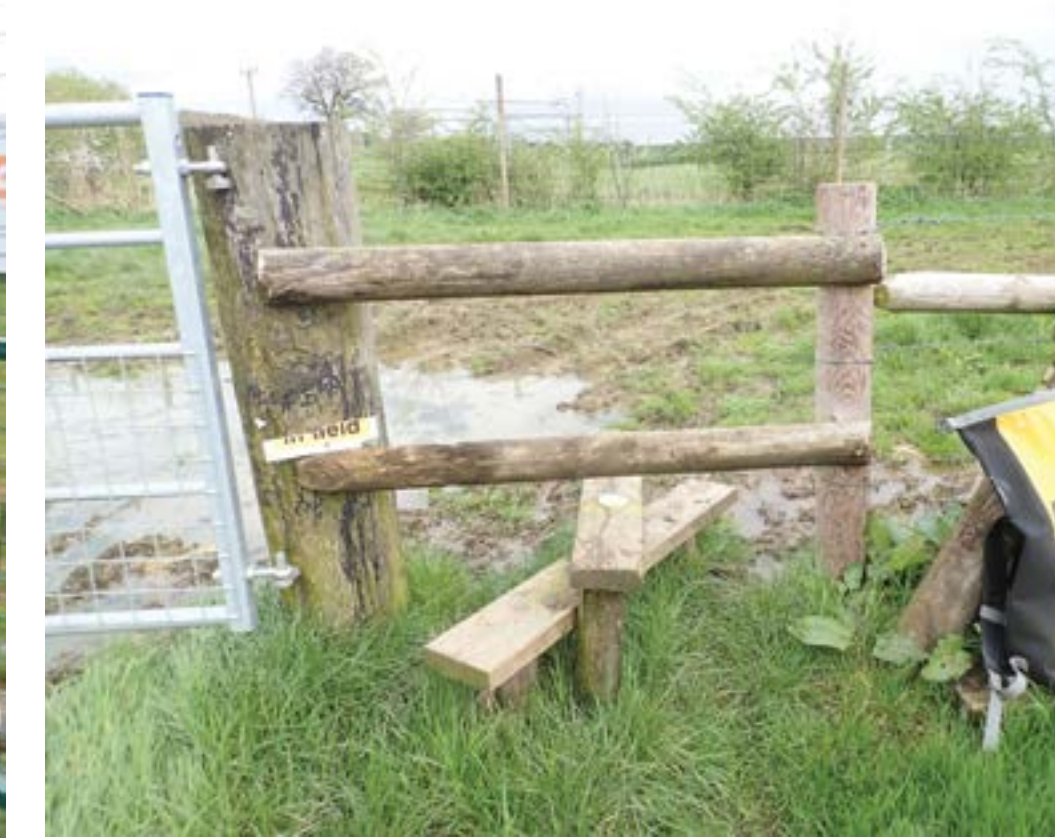
'creation of new permissive paths' Leaving walkers to find their way over rough grass around the outside of security fences while waymarkers still point to former public footpaths. (Norrington Common, Melksham, ST874647)
