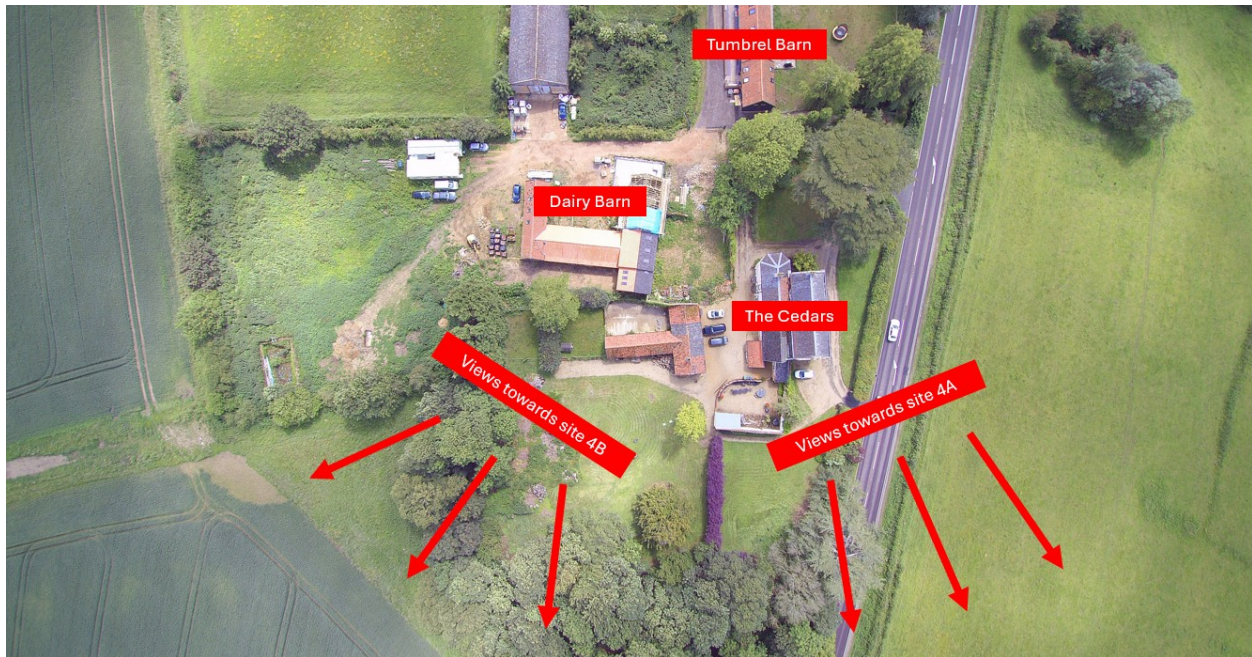
Figure A1 - Annotated aerial view of the Cedars Cluster. Red arrows indicate the general direction of views towards Sites 4A and 4B; they do not indicate the Scheme boundary.
