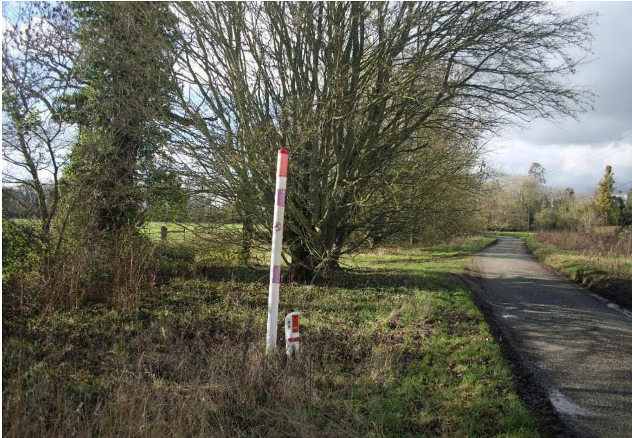
High Pressure gas mains pipe at proposed site 7F entrance on Saxlinham Green (grid ref TM2473 9646)
