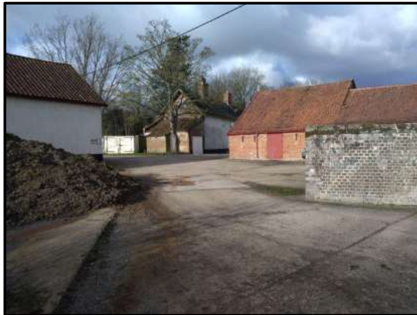
Church Farm Farmhouse, Rhee Lane: Grade II listed at the junction of Church Lane ,Stratton St Michael and Stratton Lane.
