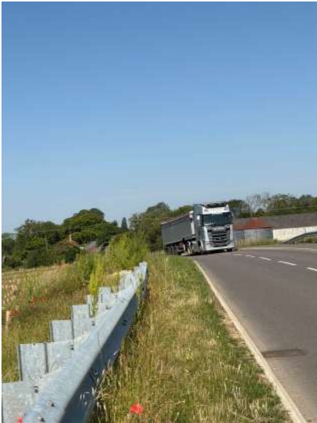
Images of Hall Lane bypass bridge showing new changed road layout which is also planned for Highway works shown in section 56 notices
