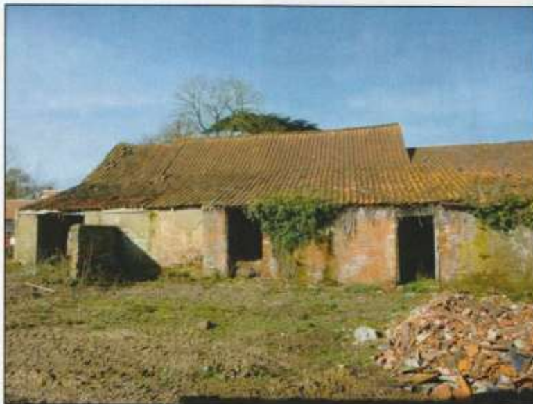
Photo 2. Dairy Barn east elevation.
