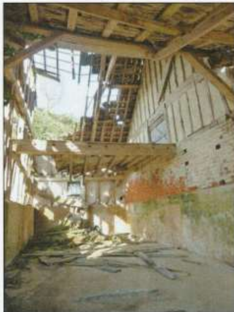
Photo 4. Interior of Dairy Barn (southern end).
