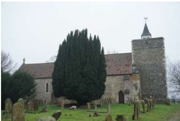
Stratton St Michael, Grade I Listed
