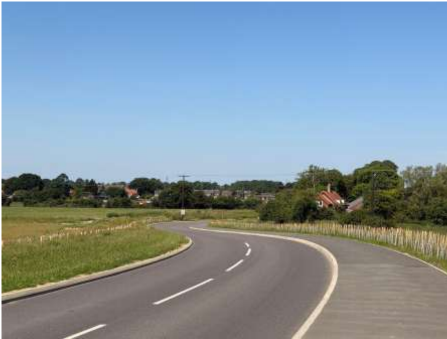
Hall Lane, Eastbound approach to bypass bridge looking west
