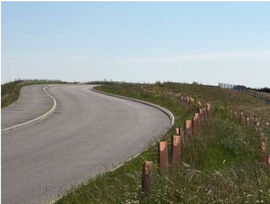
Hall Lane, eastbound approach to bypass bridge looking east
