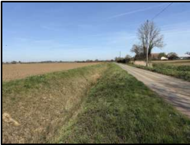
Drainage ditch at Parker's Lane 3m deep as field floods and is in EV Flood Zone
