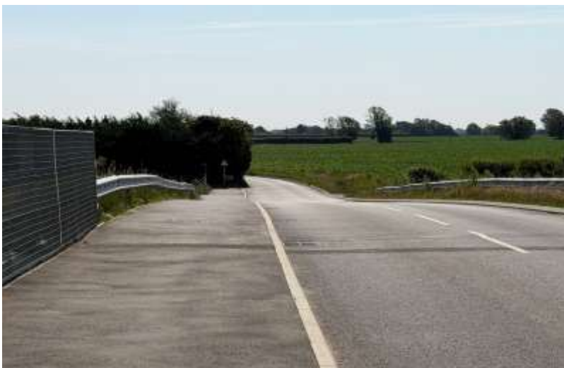
Exiting east from the bypass bridge, Hall Lane with the narrowing and blind corner at Reeves Cottage
