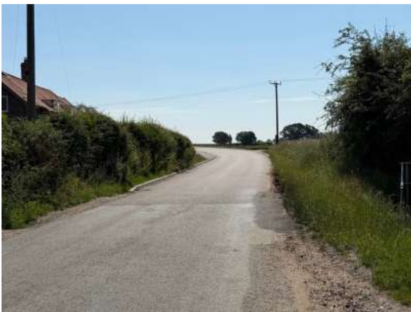
Eastbound approach towards bypass bridge, Hall Lane
