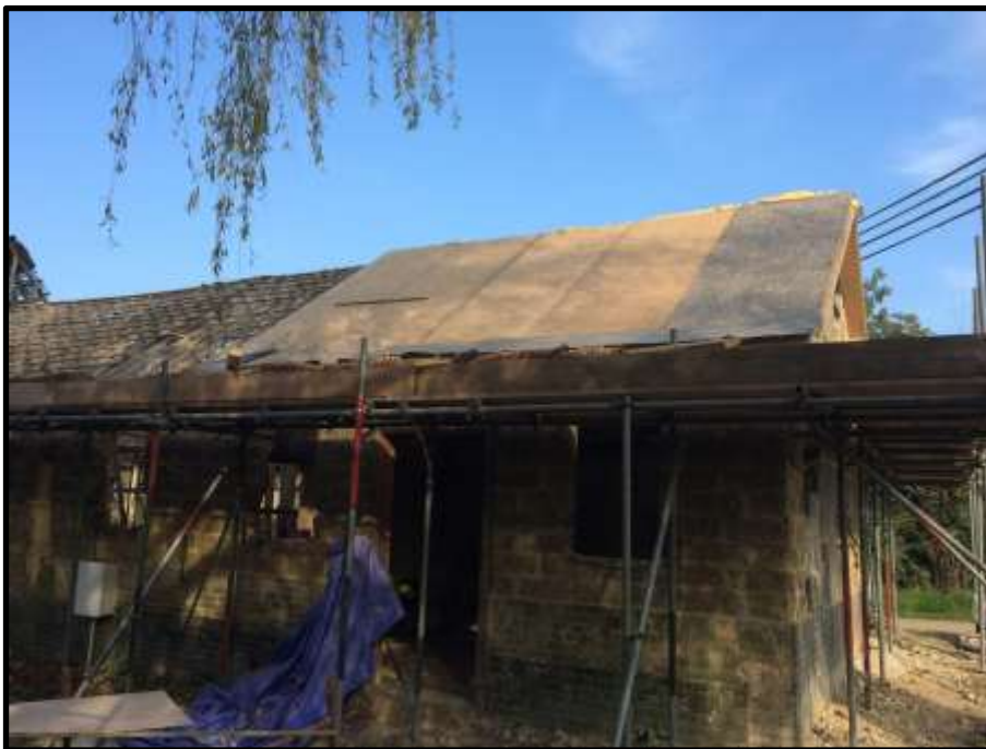
Tumbrel Barn during conversion showing the clay lump construction.
