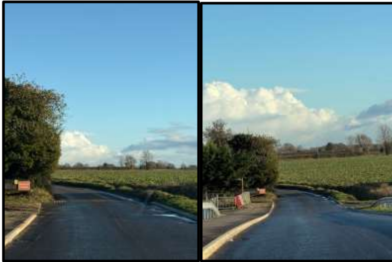
Hall Lane on the east side exiting the by-pass bridge as it approaches a blind corner at Reeves Cottage
