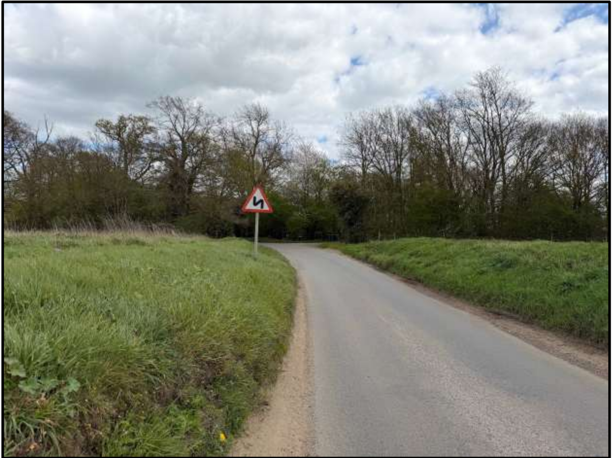
Location of Mill Lane A16 and CRC Compound 2 looking east where the visibility spay is limited as the road dips, turns and is shielded by wooded areas both sides.
