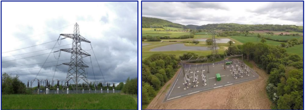
Plate 4.5 - Example of a 400 kV Sealing End Compound
