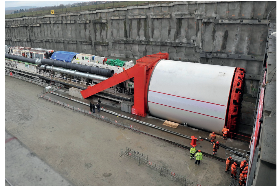
Figure 5.36: An example of the type of tunnel boring machine that would be used
