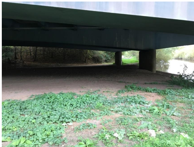
Plate 7 – Bare earth conditions created beneath the low, wide bridge B3D (H:W ratio <0.1)
