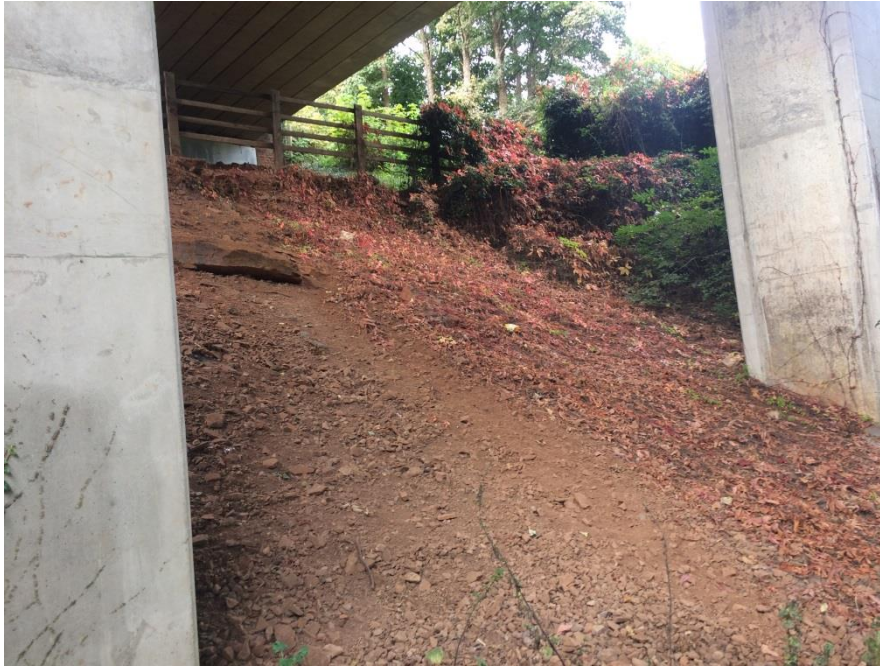
Plate 18 – Bridge B4A showing scouring of the embankments beneath the bridge
