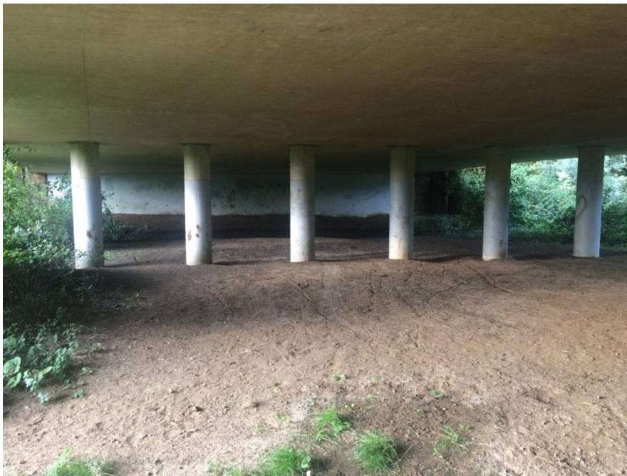
Plate 19 – Bridge B1C. A typical example of the conditions created by low height bridges
