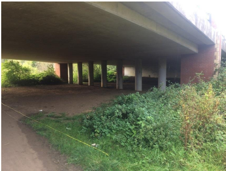
Plate 8 – Bare earth conditions created beneath the bridge B1C (H:W ratio <0.1)
