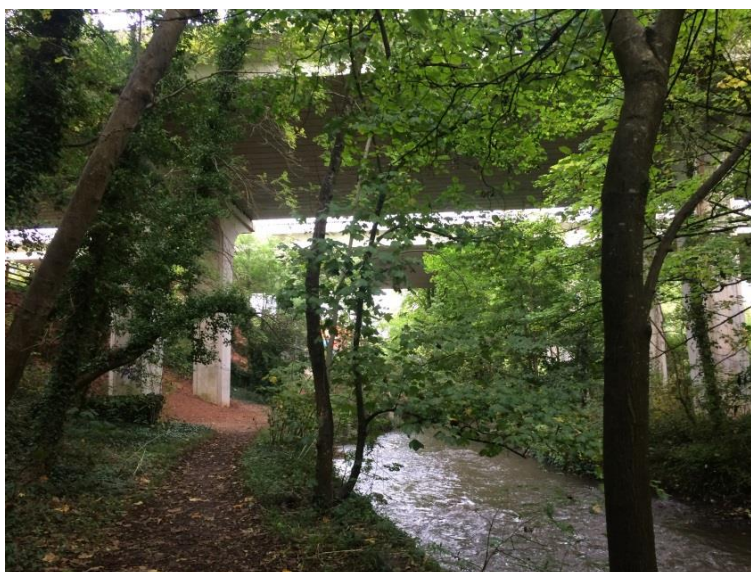
Plate 11- Extent of vegetation growing beneath and most notably within the 7m gap of twin-deck bridge B4A (H:W ratio 0.57)
