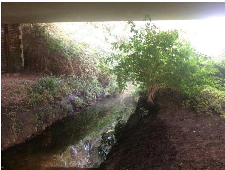
Plate 9 – Effect of shading created by bridge B1C on a small stream (H:W ratio <0.1)
