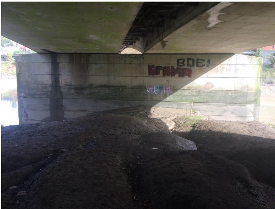
Plate 17 – Bridge B3B displaying severe scouring of the river bank
