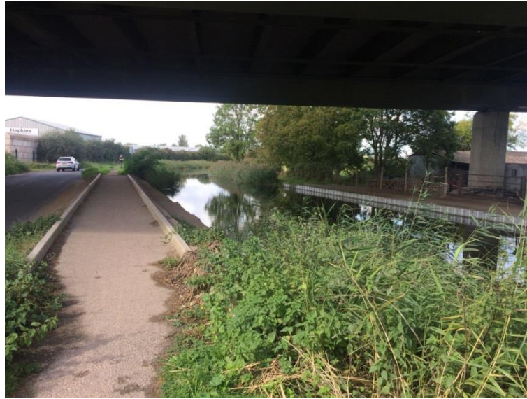
Plate 6– Dense shading and decrease in marginal vegetation beneath bridge B4E (H:W ratio 0.2)
