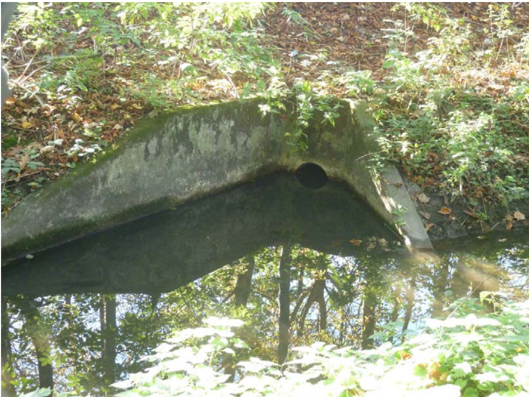
Photo 2- Additional outfall in Hollywell Brook assumed to be from the surrounding car parks.
