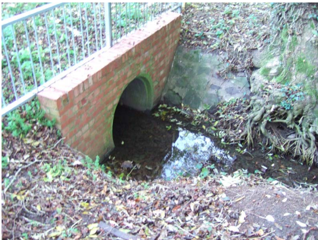
Photo 6 - Shadow Brook at the culvert (1m x 1m) crossing with Shadow Lane.
