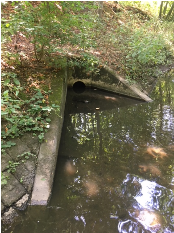
Photo 2-4 Reinforced embankment and outfall on west side of M42 of Hollywell Brook
