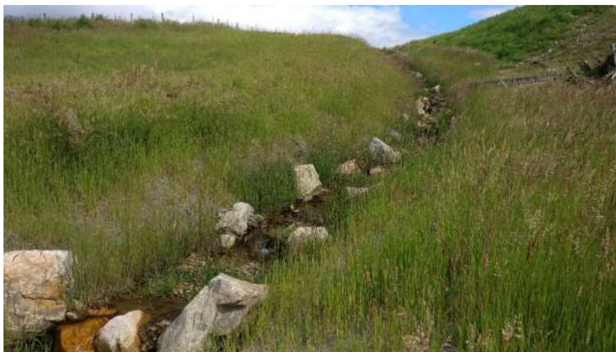
Figure 5-2 - Engineered step pool sequences on channel associated with Aberdeen Western Peripheral Road
