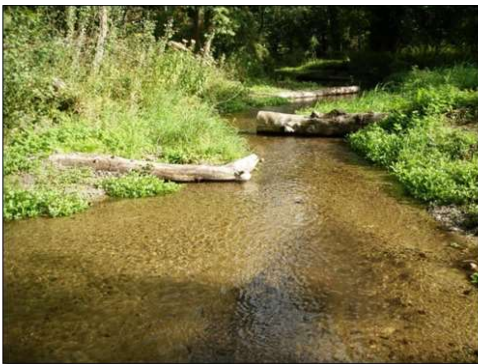
Figure 3-1 - Example of in-channel deflectors (River Wensum, Norfolk)
