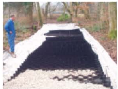
Installation of the CellWeb™ system.
