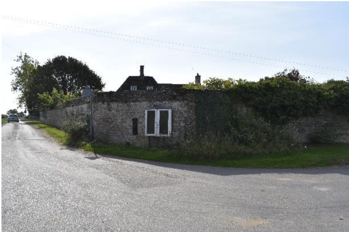
Photo 7 Model Farmhouse and wall, looking south-west
