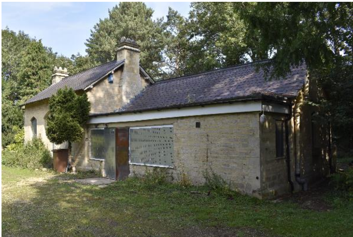
Photo 8 Former station, looking north-east
