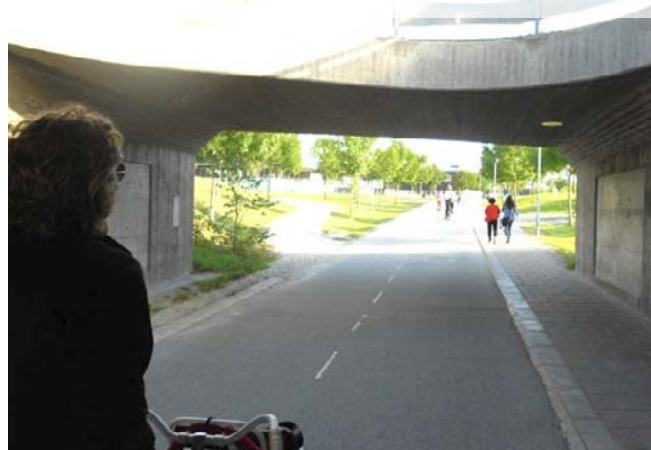
Figure: 10.52 Underbridge (cycle and pedestrian-only) with divided carriageway above to create opening – Lund, Sweden
