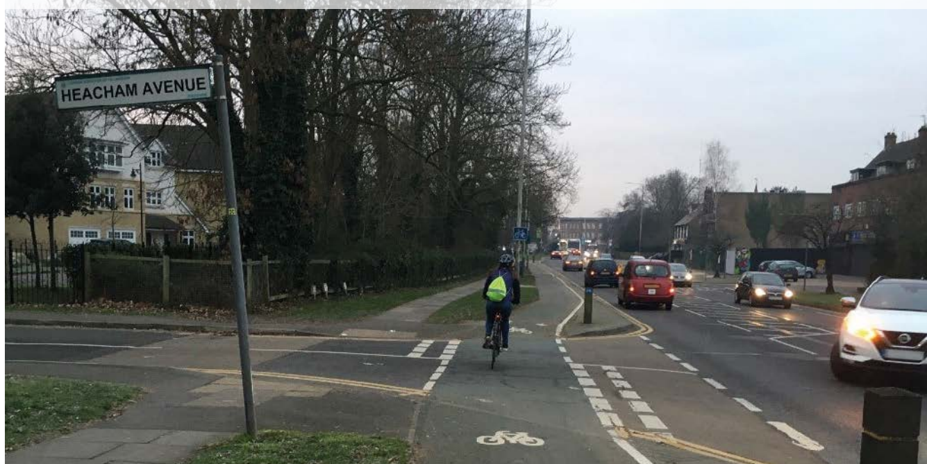
Figure 10.16: Partial set back, marked priority crossing, Hillingdon
