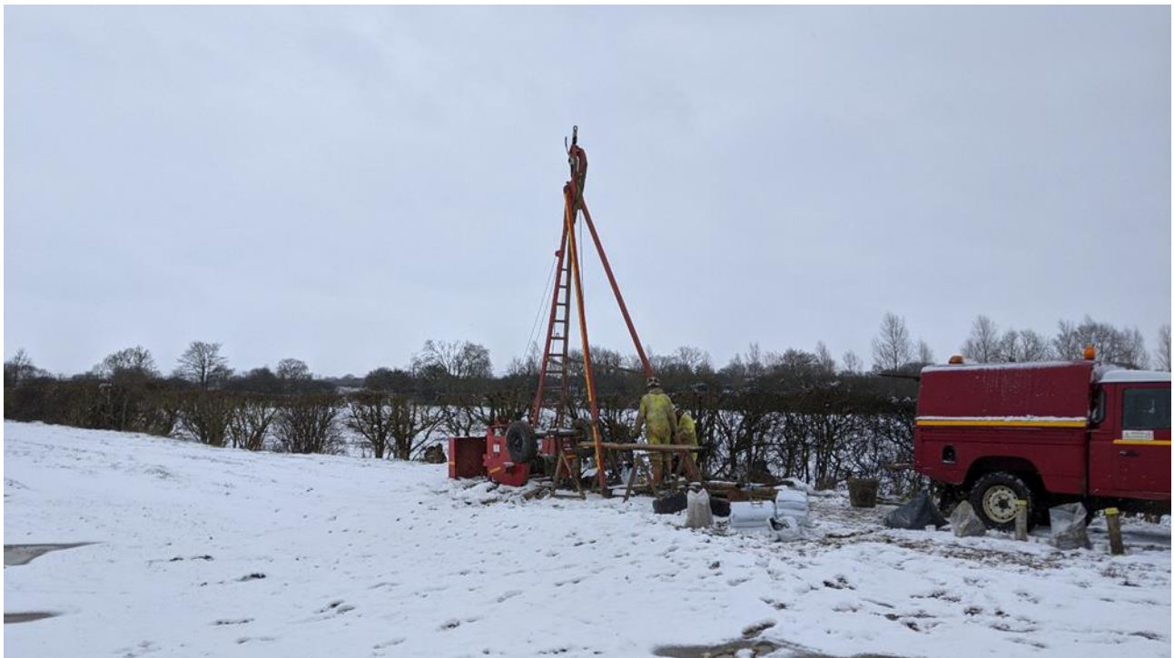
Plate 8.1 Borehole drilling during the ground investigations
