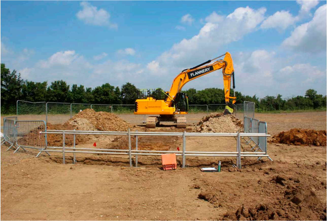
ILLUS 5 Safety set up of test pits, including an observation bridge, Herras fencing, and pedestrian fencing
