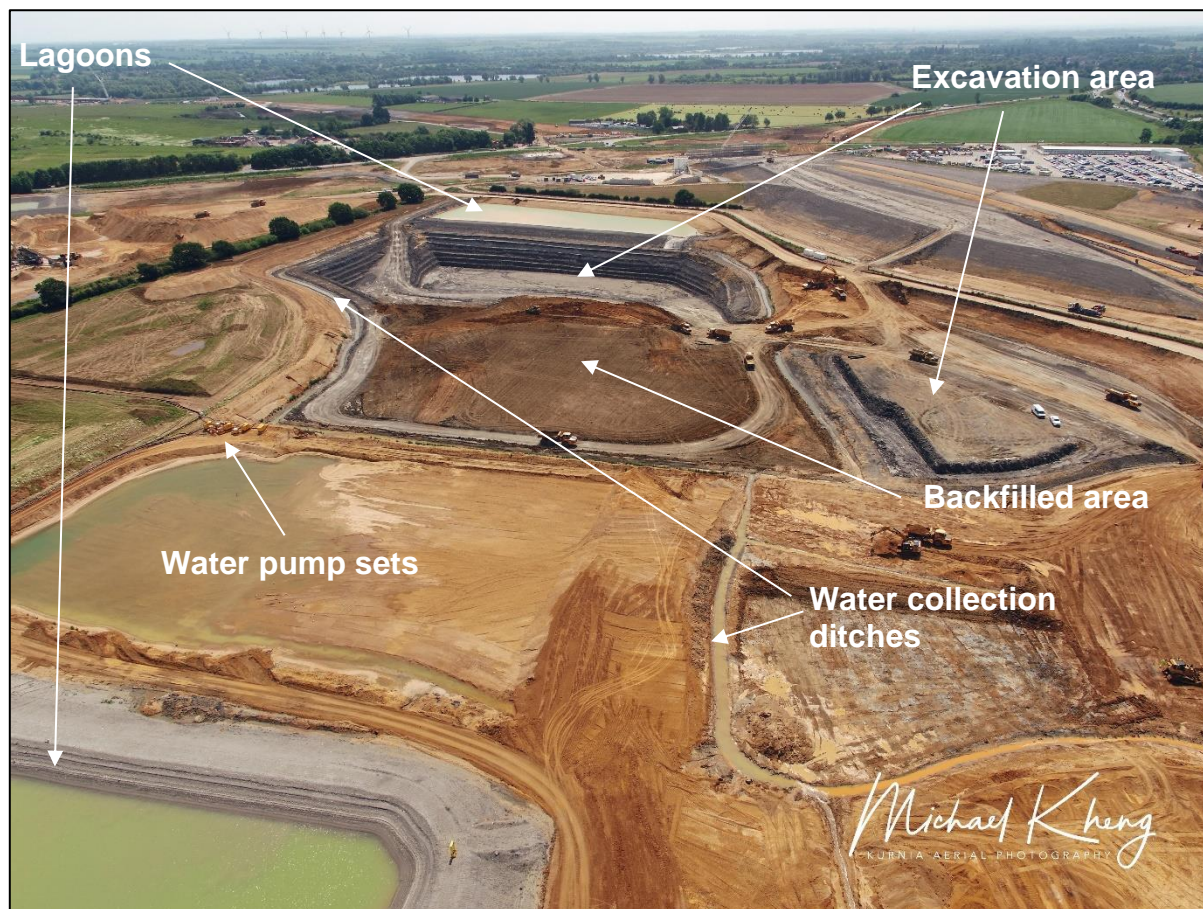
Plate 3.1 Photograph of a working borrow pit (credit: Selwood; Michael Kheng, Kurnia Aerial Photography)
