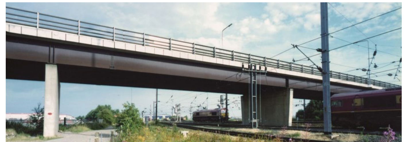
Image 7.9 Weathering Steel Overbridge (A6182 East Coast Mainline)
