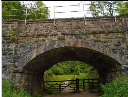
Photo 21. S026 Nightingale Valley underpass is a typical example of the small, relatively well maintained brick arches for access under Portbury Freight Line
