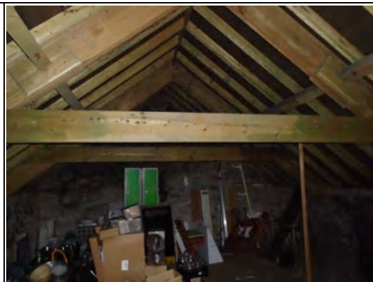
Photo 30. Lodway Farm Building LF7 – the interior of the barn shows the new roof structure. Date: October 2018
