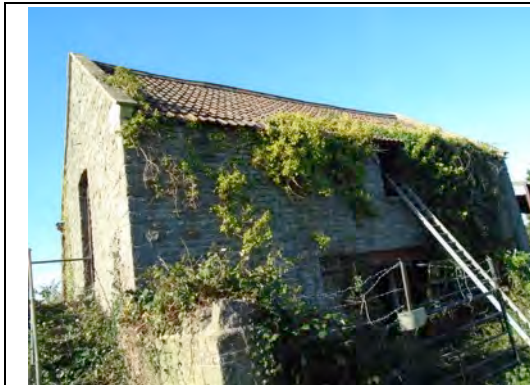
Photo 23. Lodway Farm Building LF1 – the exterior walls are solid and without crevices.
